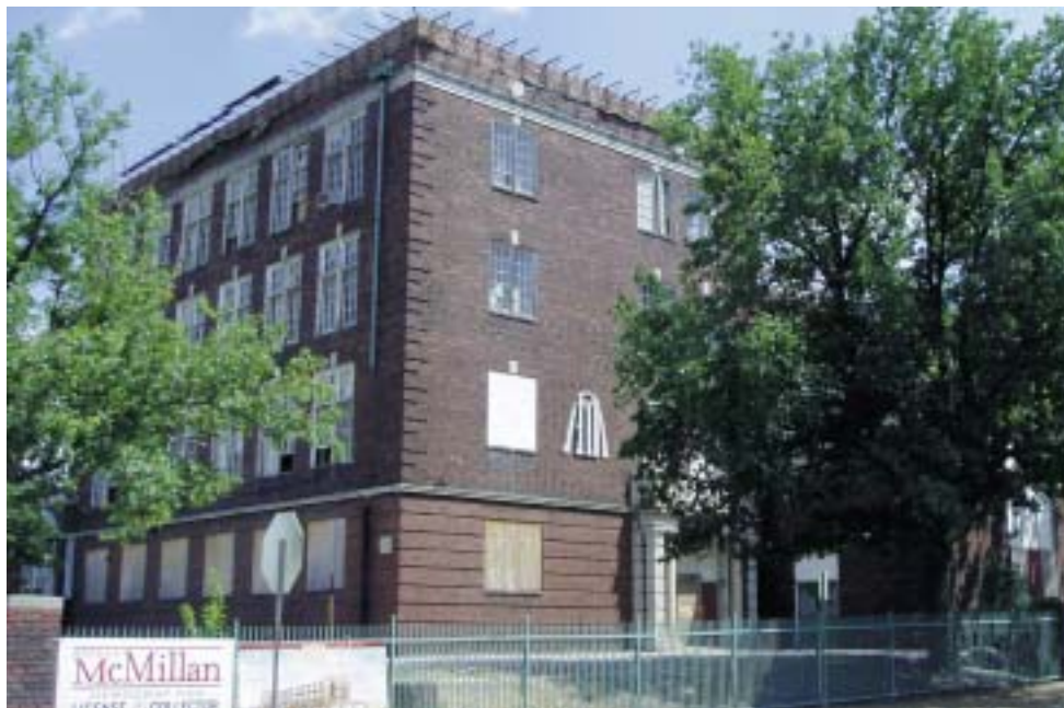
Franklin School Apartments under construction
