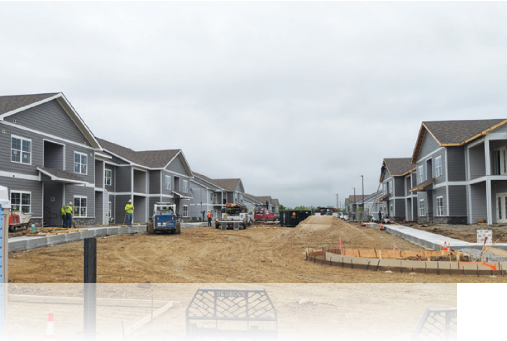
Windridge Estates II construction photos
